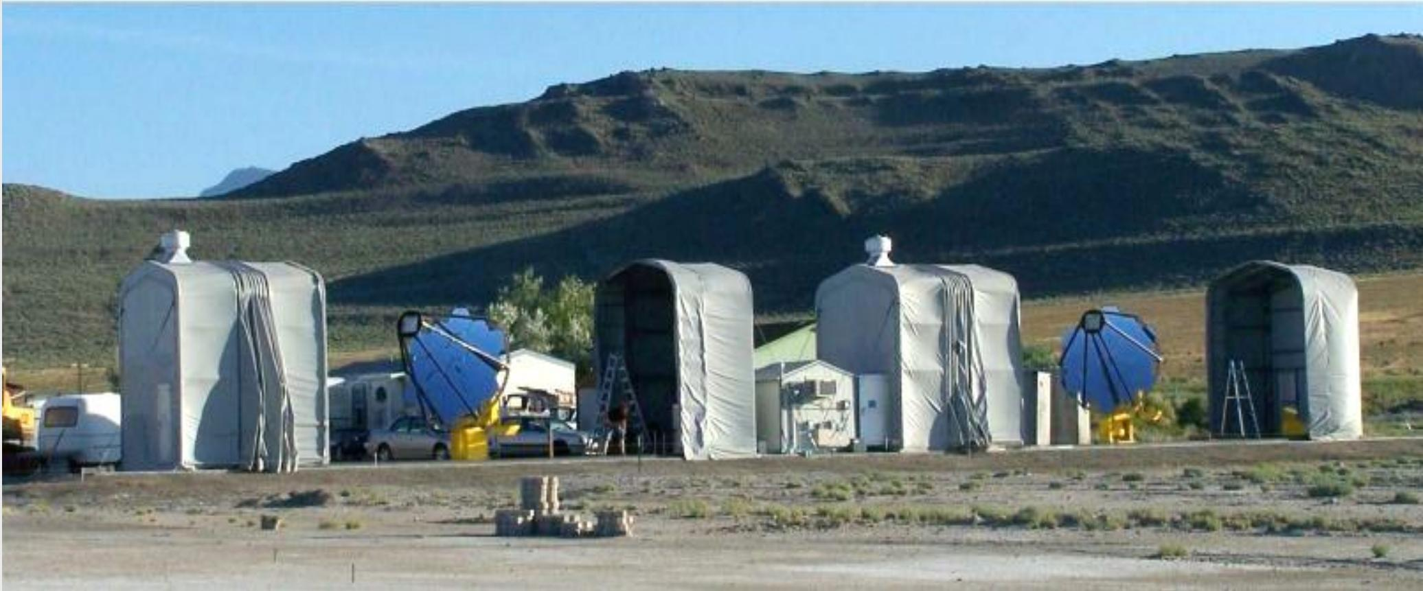
The StarBase 3 m Cherenkov telescopes are protected by buildings which can be rolled open for observation. The control room is located between the two telescopes.
